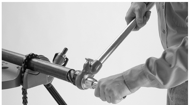
Figure 4 – Reaming End Of Pipe
