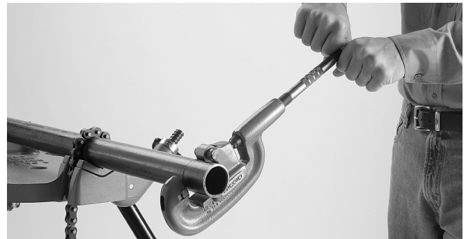
Figure 3 – Cutting End Of Pipe
